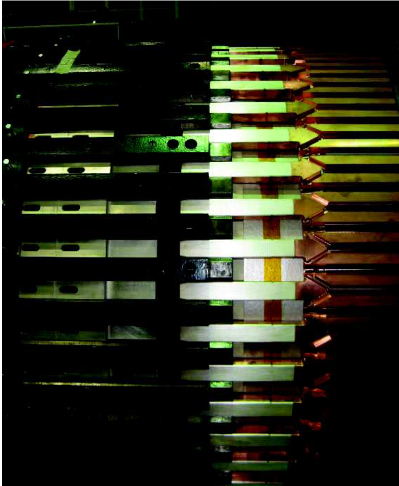
Figure 6: Reassembly of damper basket NDE, silver-coated damper fingers slide to the left on top of silver-coated damper bars
